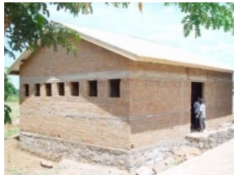
The New Sanitation Block
